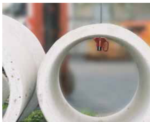
Once set, you are ready to lift the pipe.
