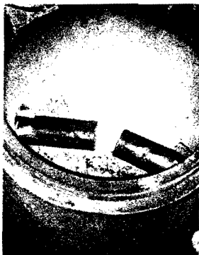
Placing Flowline Tubes
