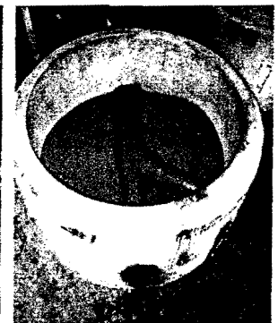
Finished Manhole Base complete with Dura-Seal Gaskets
